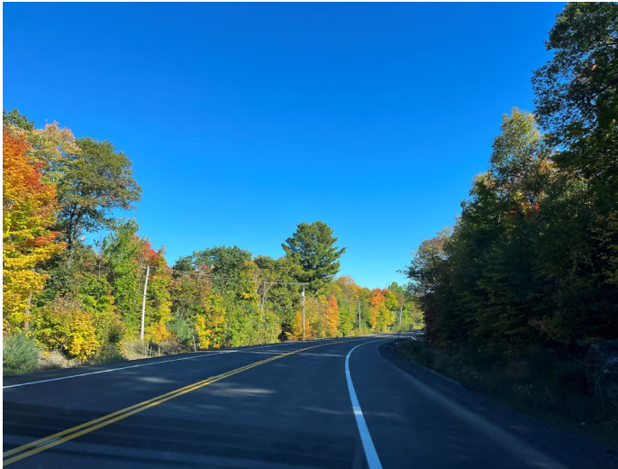
Paved Shoulder on District Road 169
