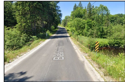
Location: Bridge Along Beatrice Townline Road (Source: Google Streetview)
