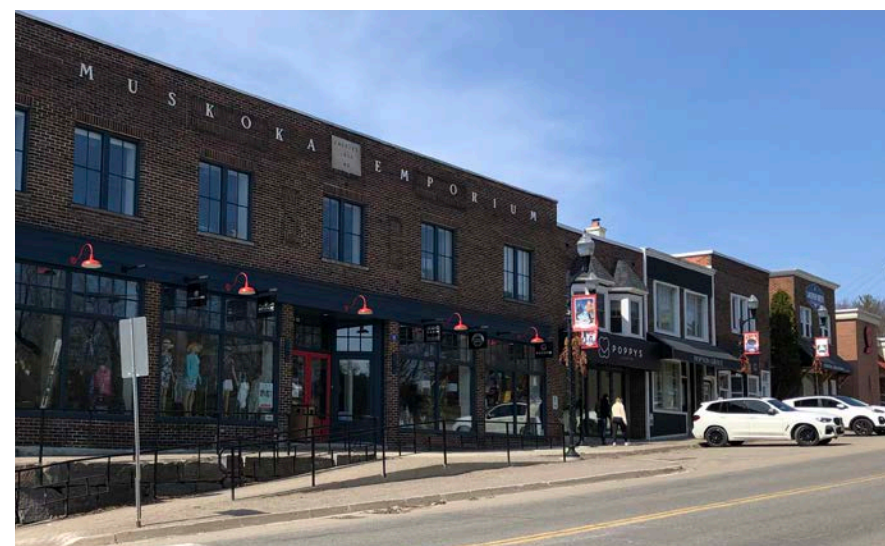
Street wall of the main street buildings on the west side of Maple Street
