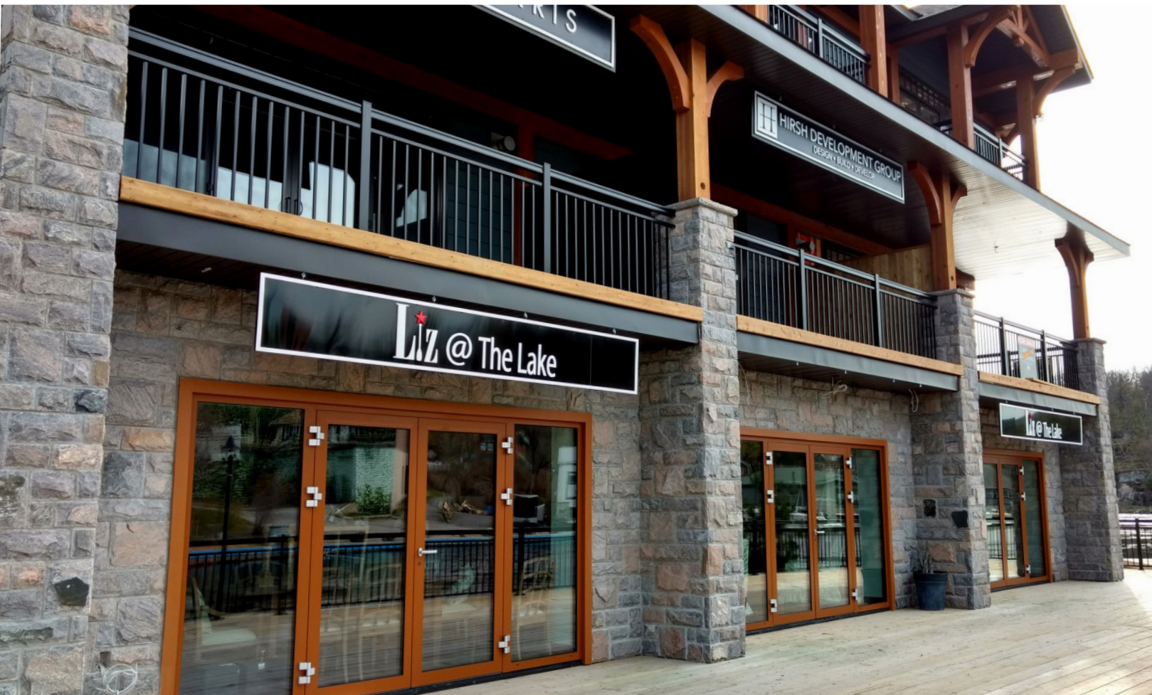
Example of a new development using Muskoka Style elements in Port Carling
