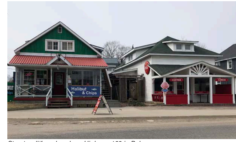
Street wall/facades along Highway 169 in Bala
