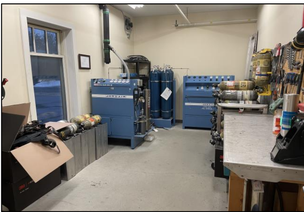
Breathing Apparatus Filling Station
