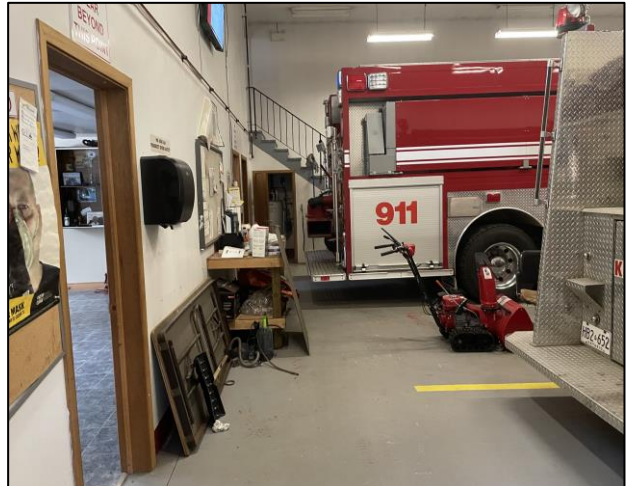
Door left open and exposed to diesel exhaust
