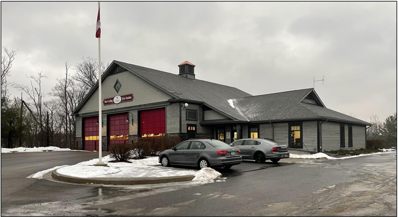
Rear of Station
