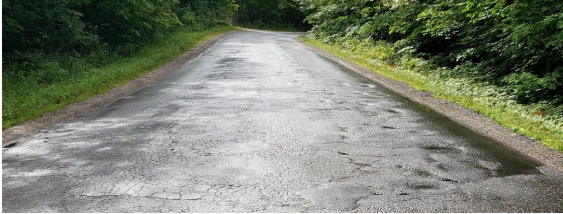
Figure 15: Example of Road Segment in Poor Category (Condition Rating 2.0 to 3.9)
