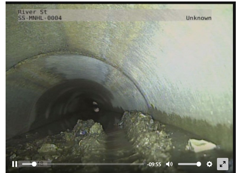
Figure 25: Fair Condition Heavily Silted In, Fair Structural Condition with Minor Defects (CR=5.5)
