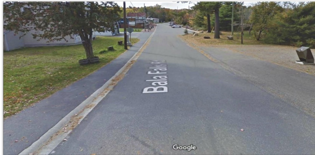
Figure 12 Example of Road Segment in Very Good Category (Condition Rating \geq 8.0 )
