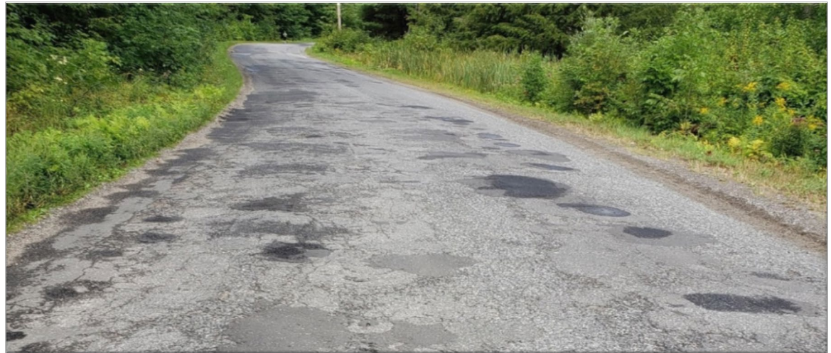
Figure 16. Example of Road Segment in Very Poor (Condition Rating <2.0)
