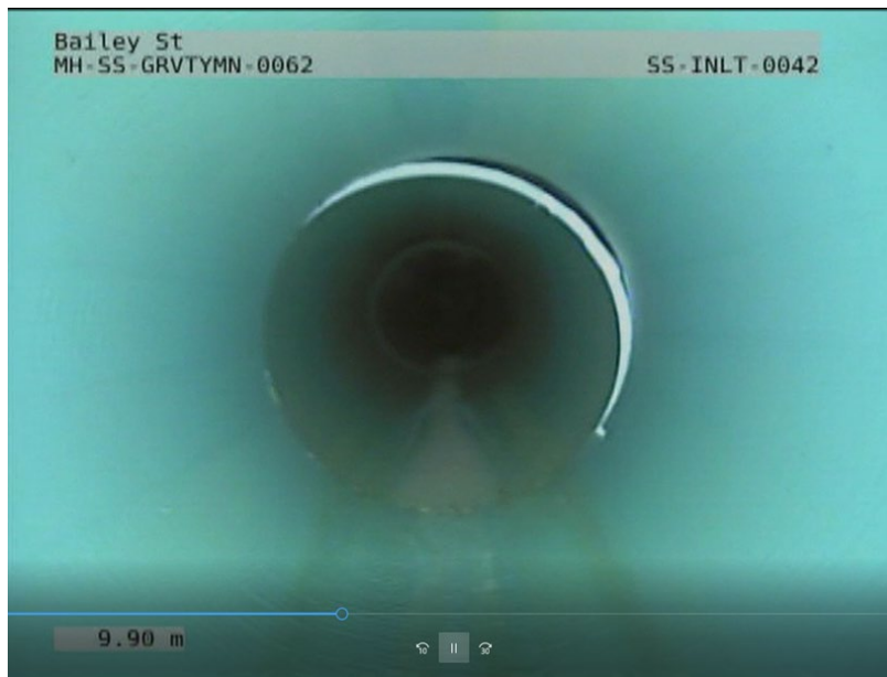
Figure 26: Poor Condition Joint Separation or Structural Failure of the Pipe, Pipe Distortion (CR=4.5)
