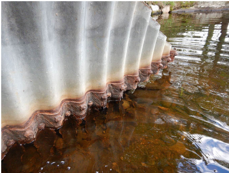
Figure 9: Dark Bay Road Culvert; Poor Condition, BSI < 40
