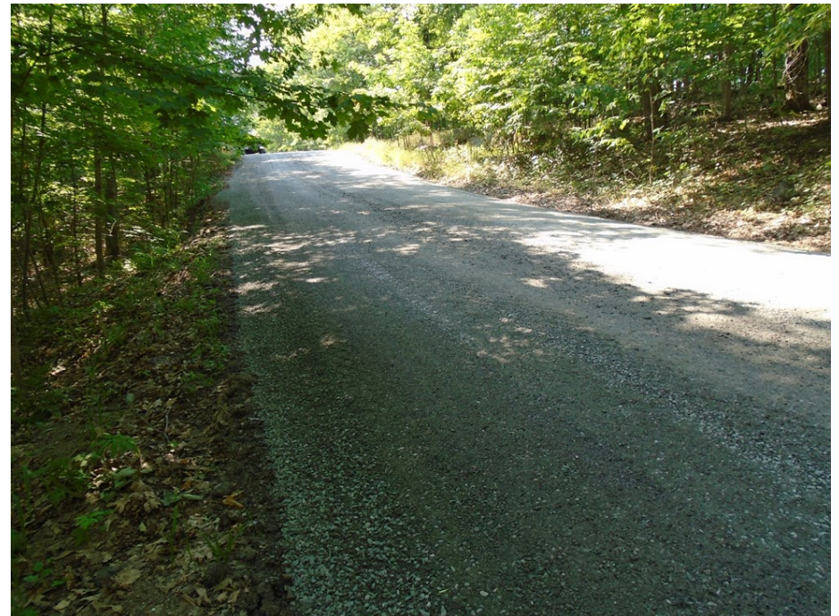
Figure 29: Good Condition: Drainage Generally Directed Away From the Road Definition of Drainage Channels Requires Improvement (CR =6.5)
