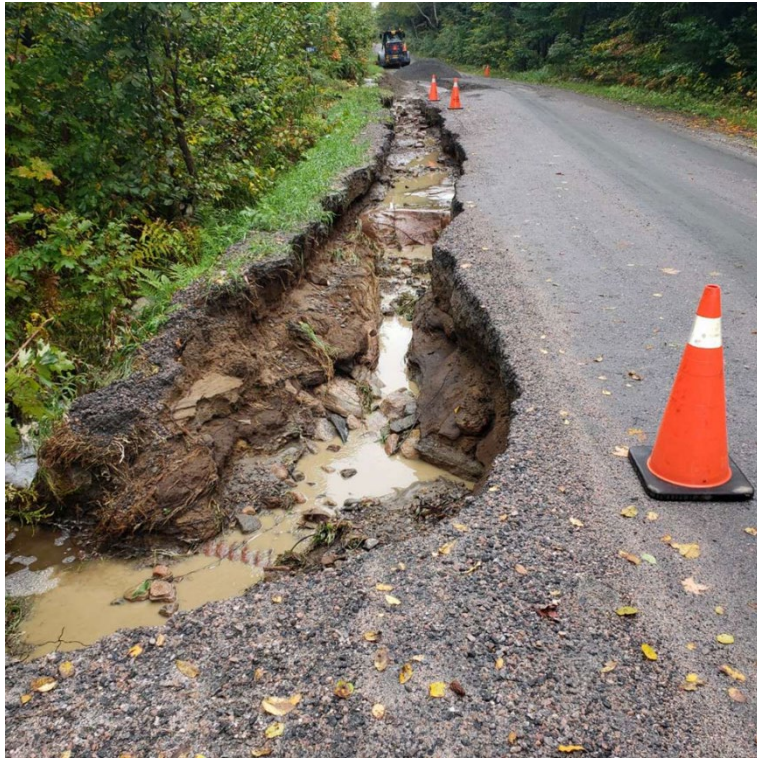
Figure 30: Poor Condition: No Defined Drainage System and Failure of the Drainage Infrastructure (CR =3.5)
