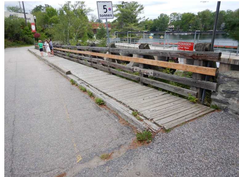
Figure 8: Bala Falls Road Bridge, Fair to Poor Condition BSI 43.6
