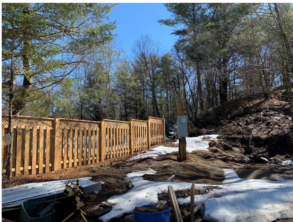
Figure 6. View of fence abutting the enclosure and storage containers.
