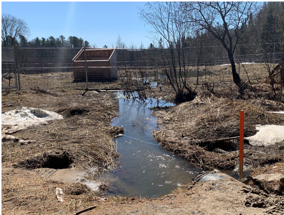
Figure 13. Stream leading to the wetland zoned EP1 on the subject property, and the moose enclosure.
