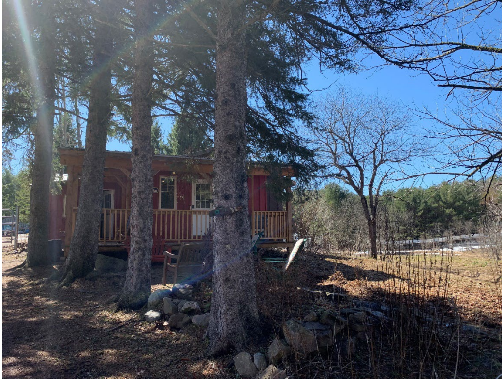
Figure 7. Existing dwelling/office identified as Building #1 on the submitted site plan.
