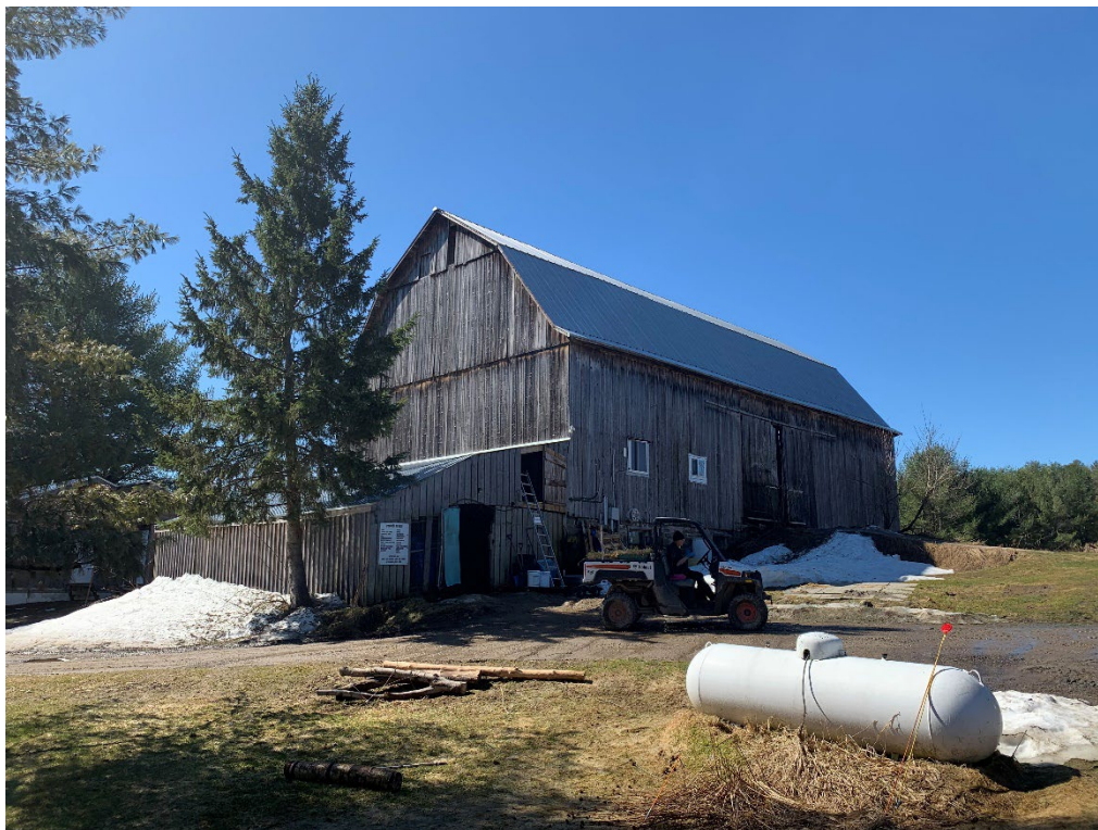
Figure 8. Existing barn identified as Building #5 on the submitted site plan.
