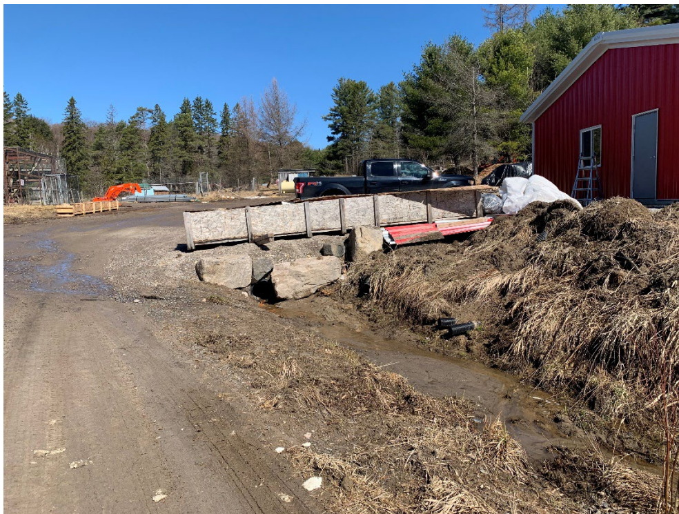
Figure 10. Stream/drainage swale abutting the recently constructed storage shed.
