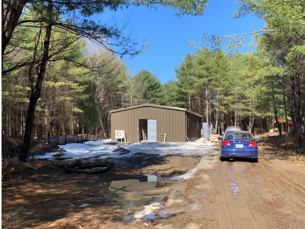
Figure 11. Recently constructed storage building identified as “storage under construction 28 x 34” on the submitted site plan.
