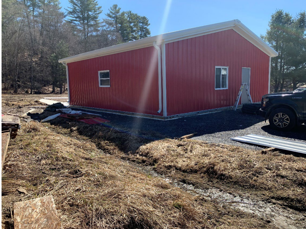
Figure 9. Recently constructed shed identified as “storage under construction 34 x 36” on the submitted site plan.
