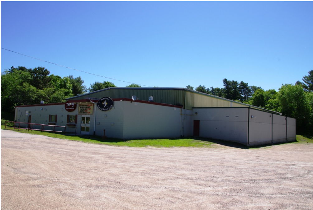
Photo 1 - West (Front) Elevation (South – West Corner)
