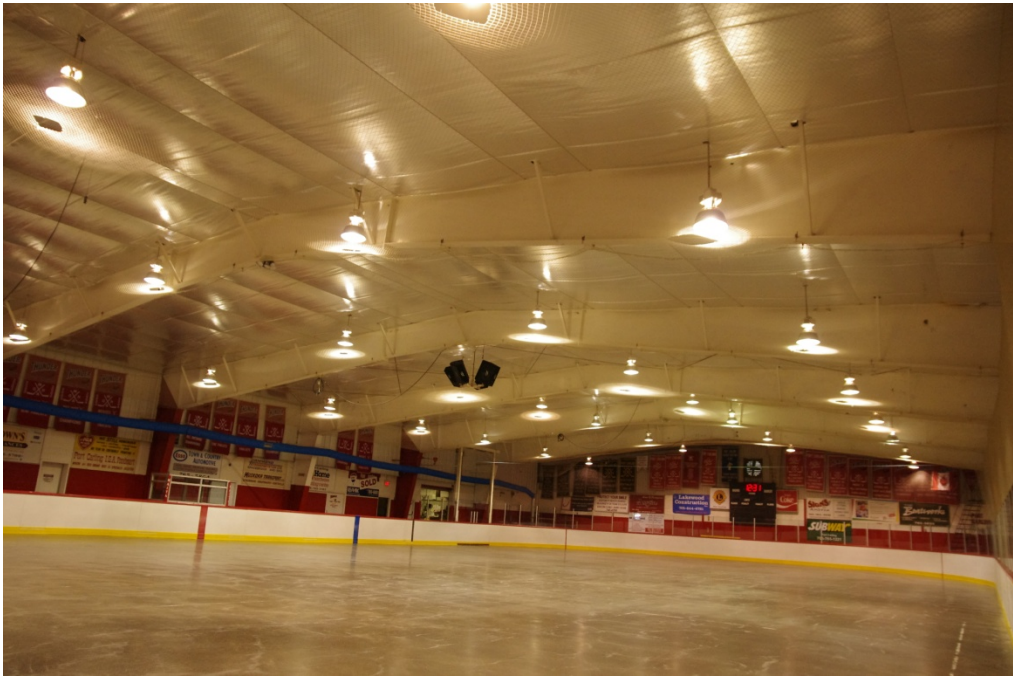
Photo 11 – Interior of Arena with Low E Ceiling below Roof Purlins
