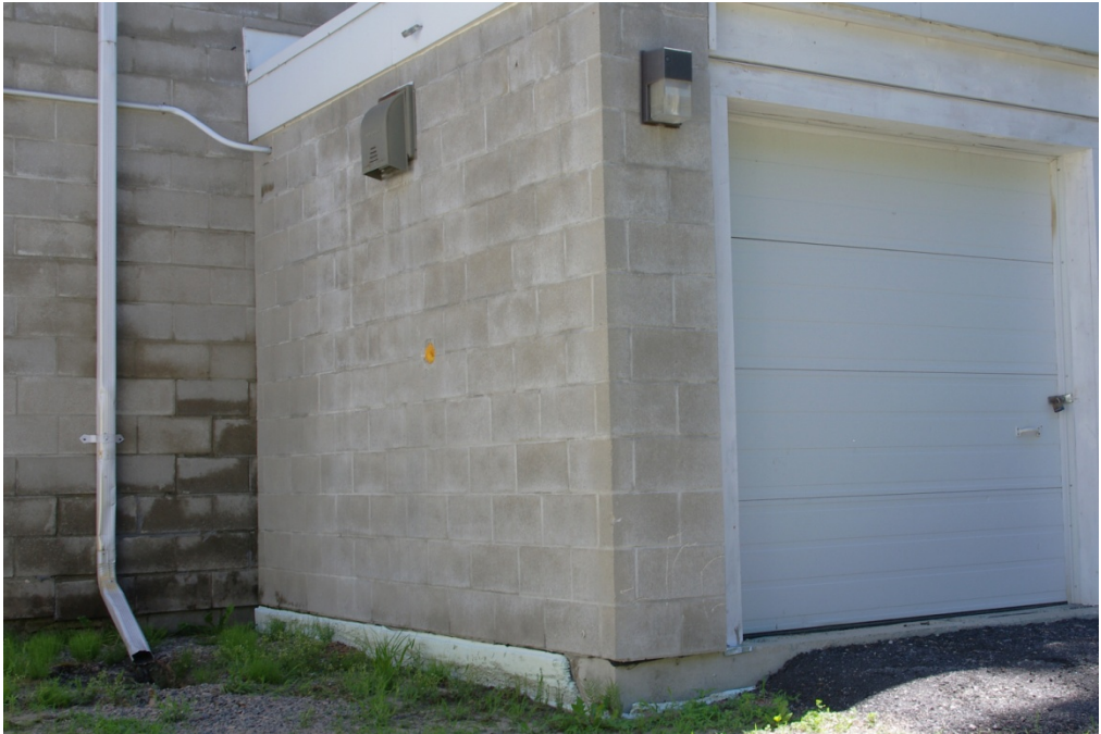
Photo 5 – Zambonie Room – Exposed Rigid Insulation
