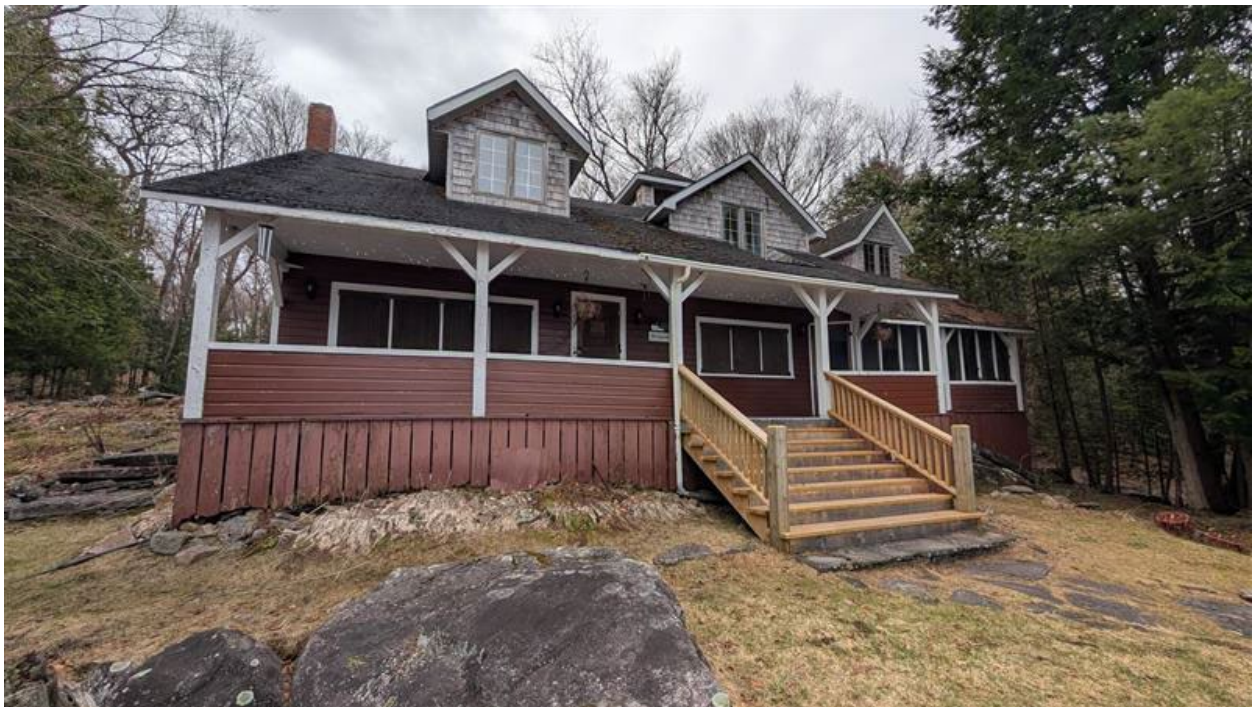
Figure 5: Dwelling on Resultant Lot 2.
