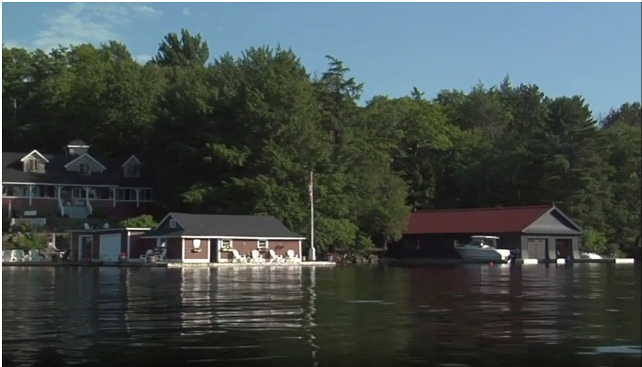
Figure 6: Shoreline structures on Resultant Lot 2 (image from Muskoka GeoHub shoreline videos)
