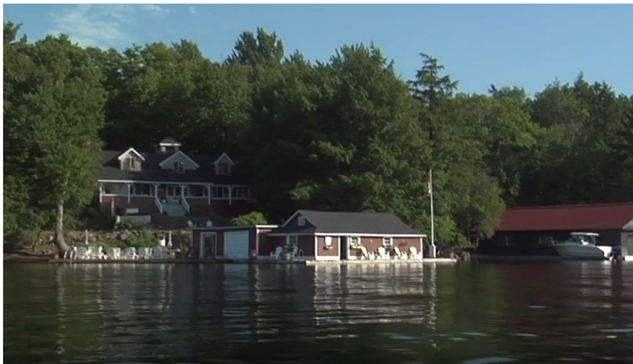
Figure 7: Shoreline structures on Resultant Lot 2 (image from Muskoka GeoHub shoreline videos)
