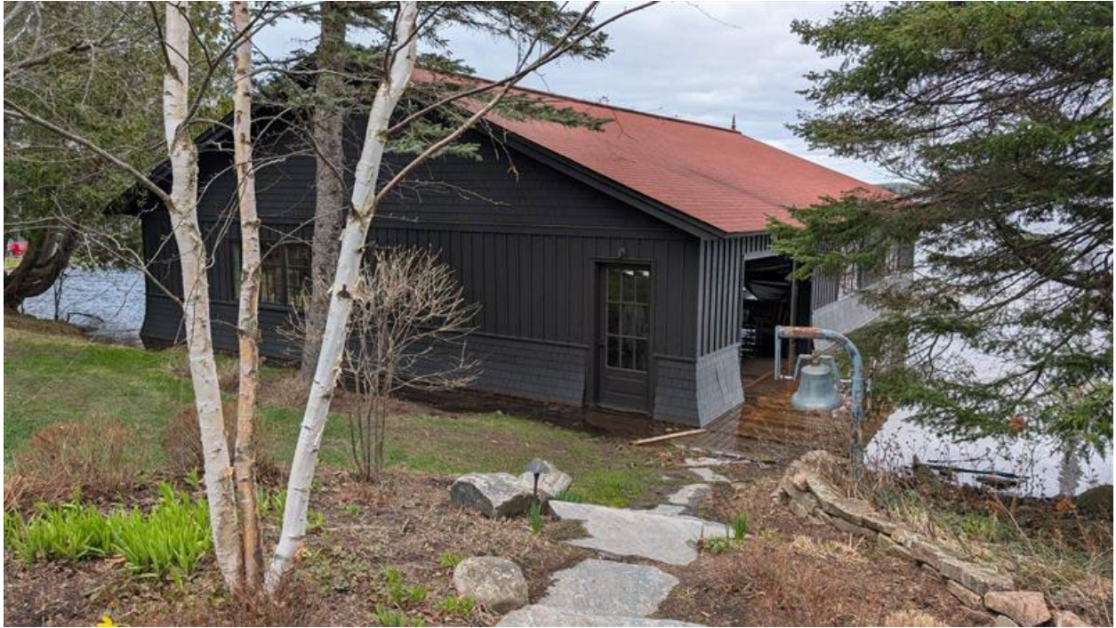
Figure 2: Boathouse on Resultant Lot 1.
