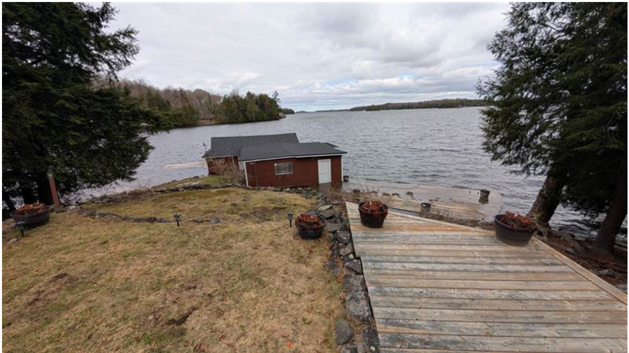
Figure 3: Boathouse on Resultant Lot 2.
