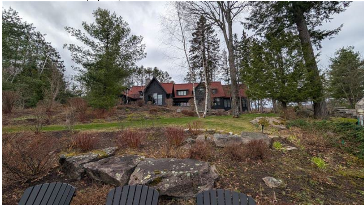
Figure 1: Dwelling on Resultant Lot 1.
