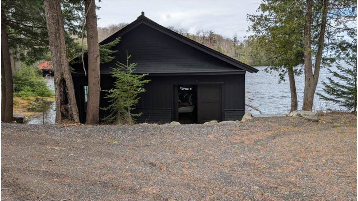
Figure 4: Boathouse on Resultant Lot 2.
