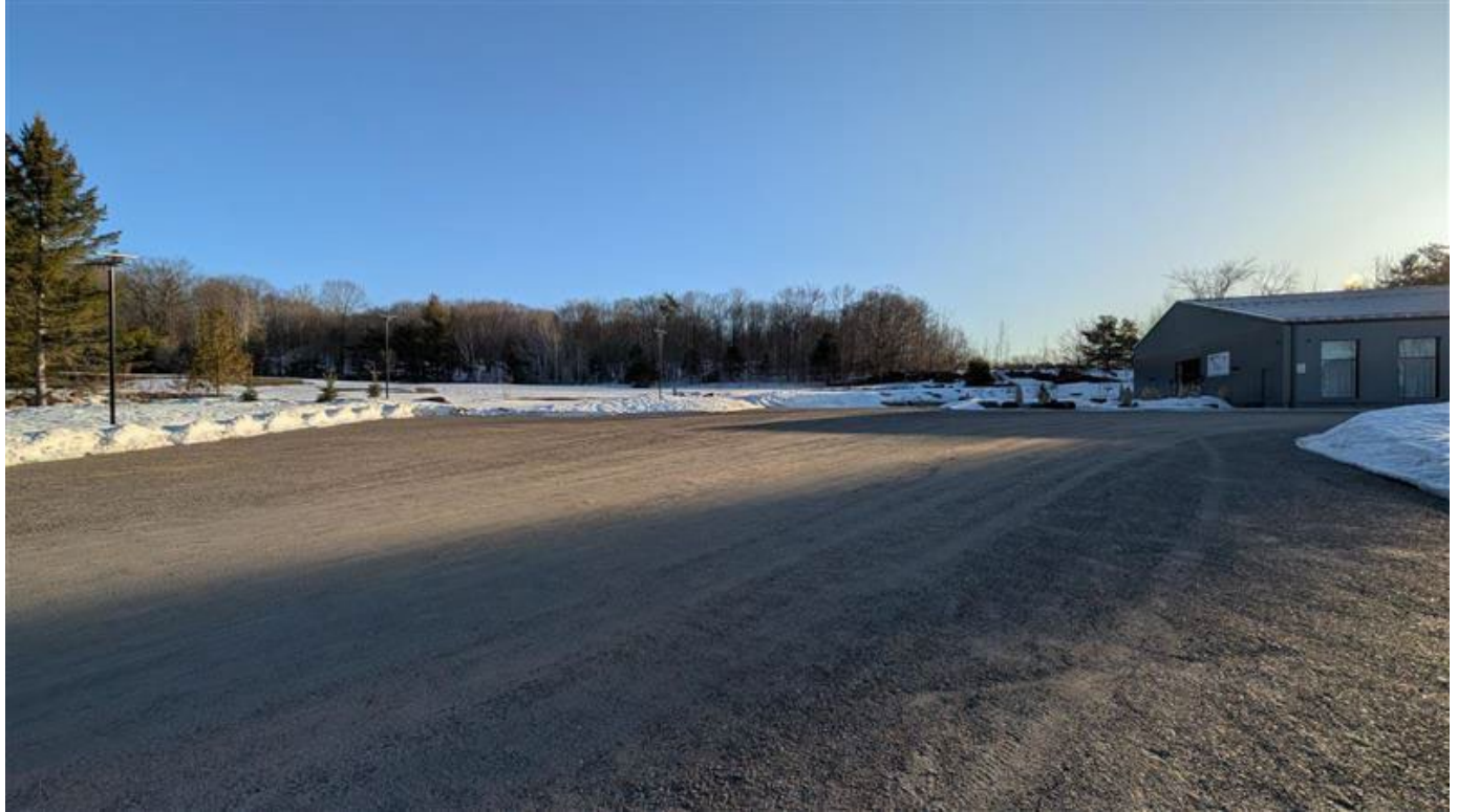
Figure 7: Parking spaces that encroach into buffer.
