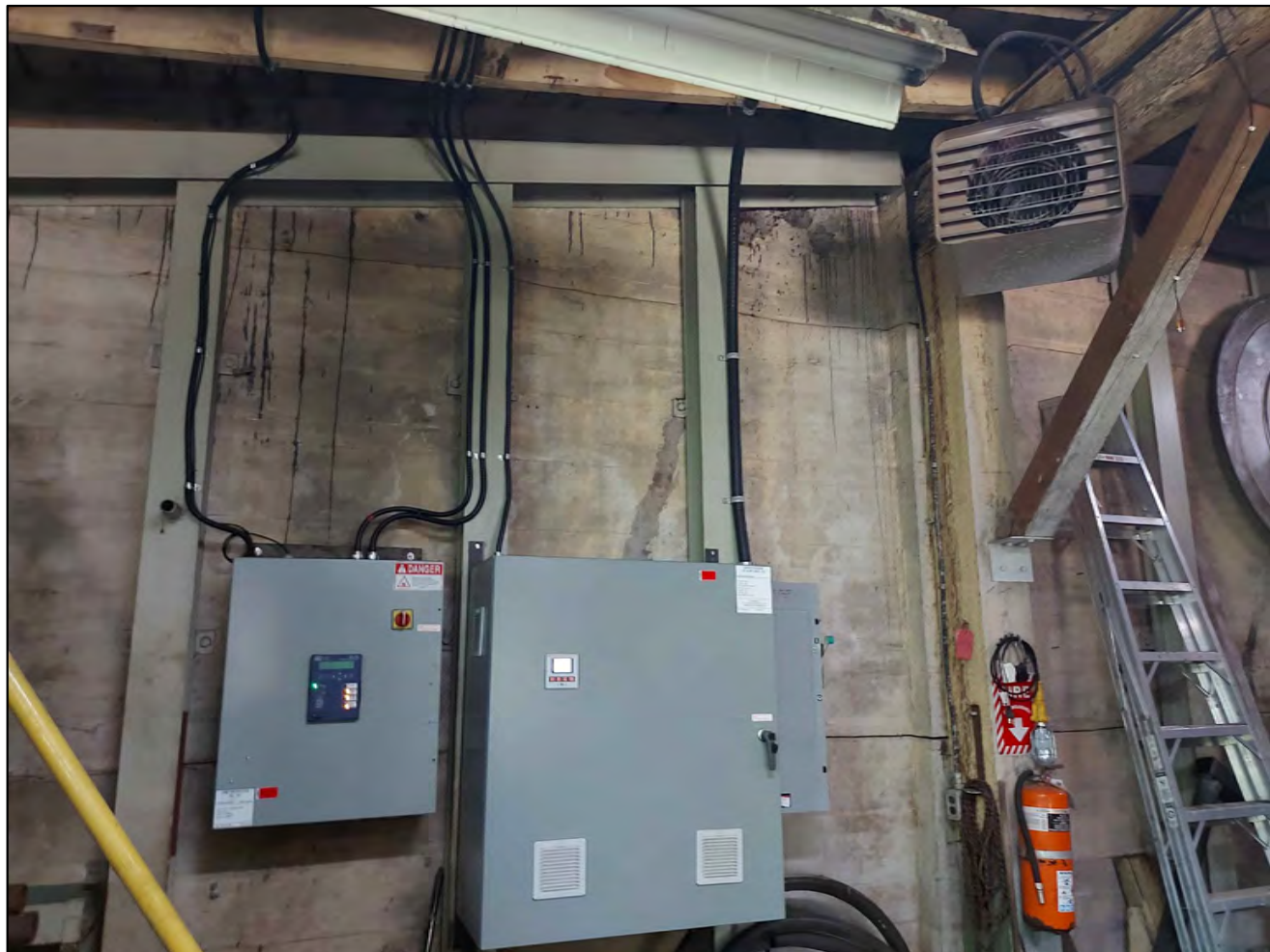
PHOTO 7 EXISTING STEELWORK -- NORTH WALL
