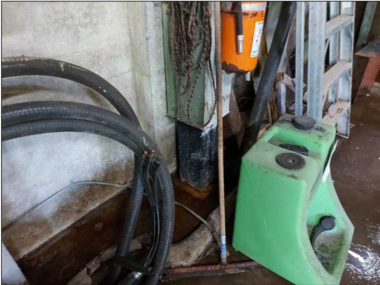
PHOTO 6 EXISTING STEEL COLUMN BASE -- NORTH WALL
