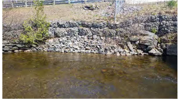
Photo H – Gabion baskets and placed boulders on the right downstream bank downstream of the dam
