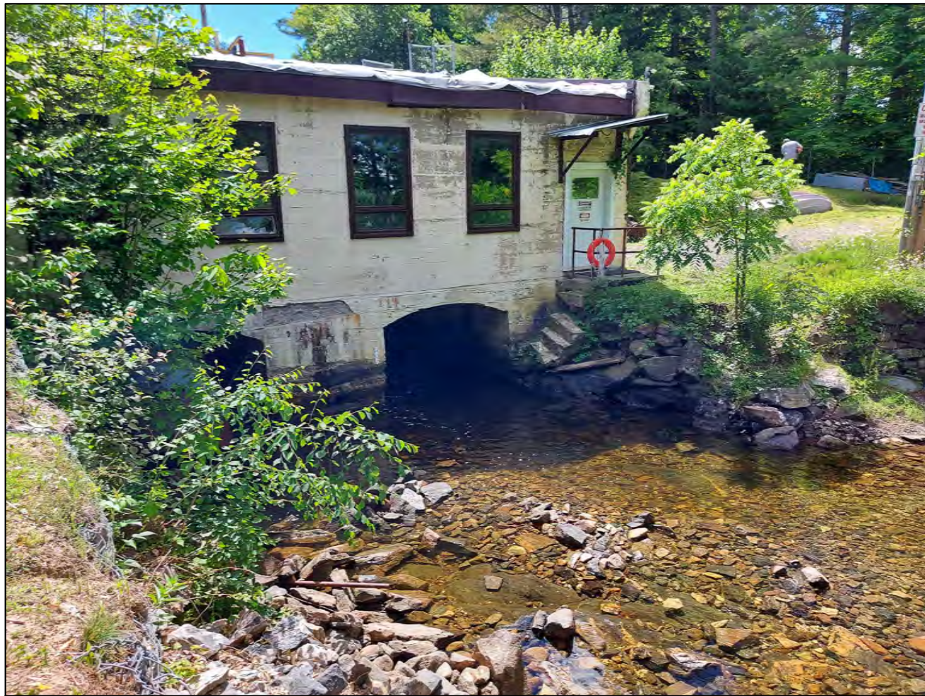
PHOTO 1 DOWNSTREAM SIDE WEST ELEVATION LOOKING EAST
