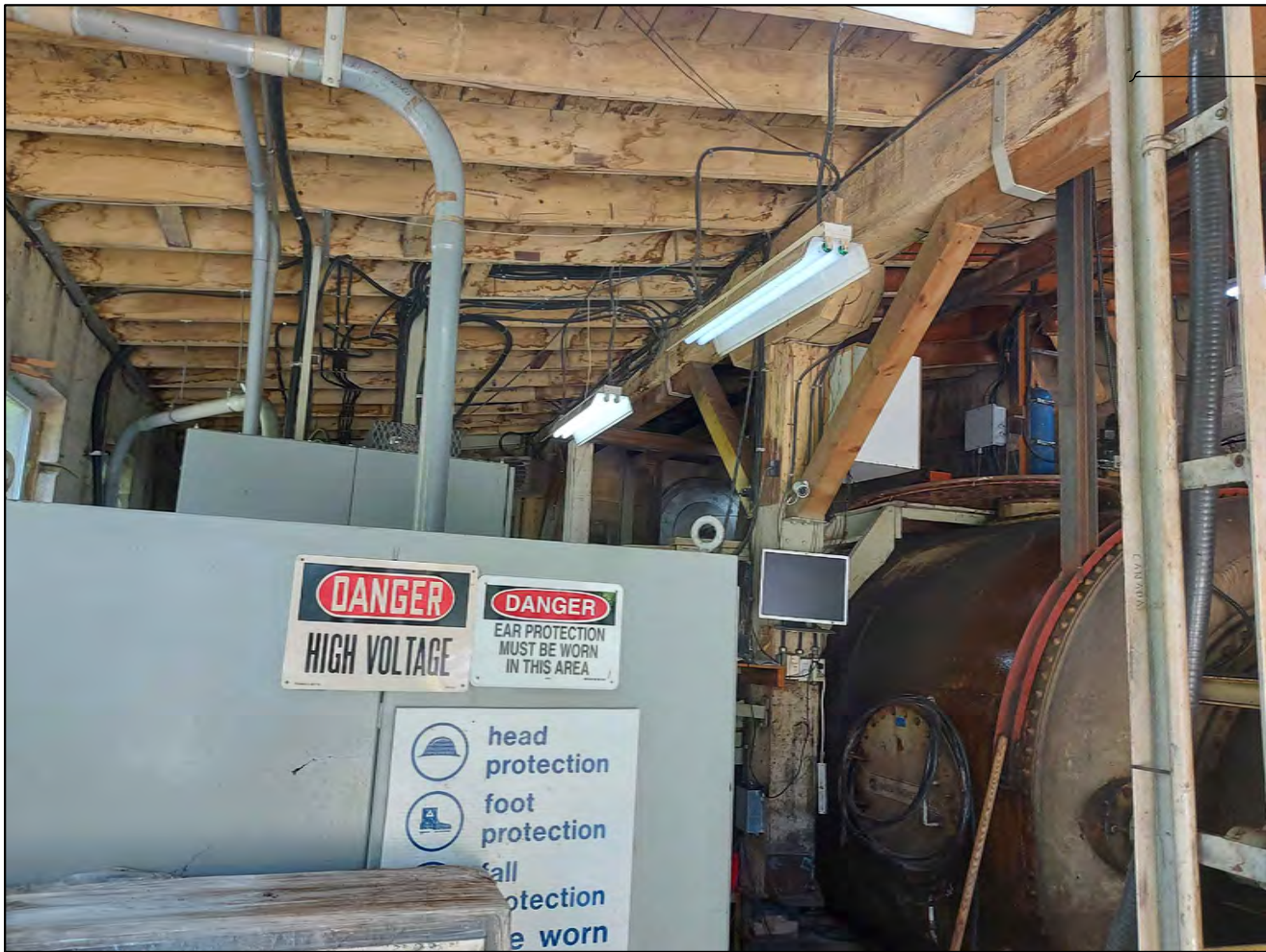
PHOTO 3 EXISTING BEAM AND ROOF STRUCTURE
