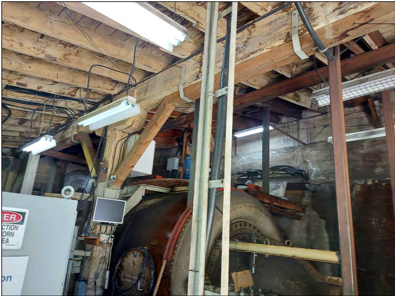
PHOTO 2 EXISTING BEAM AND ROOF STRUCTURE
