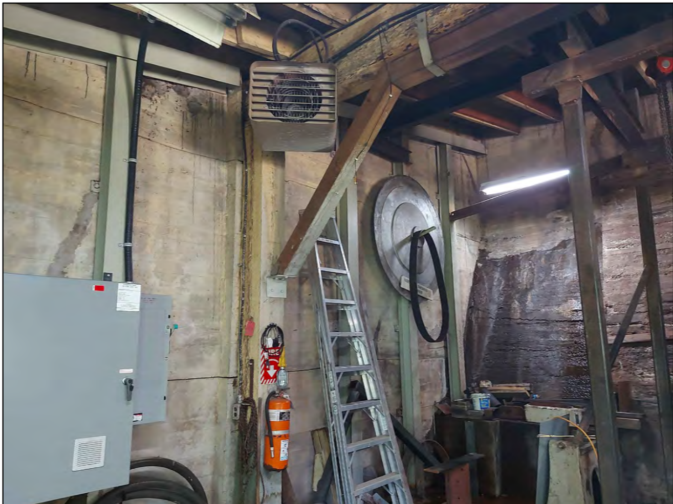
PHOTO 8 EXISTING STEELWORK -- NORTH WALL
