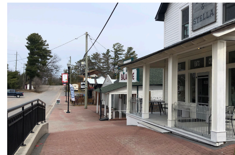
Street wall/facades along Bala Falls Road in Bala
