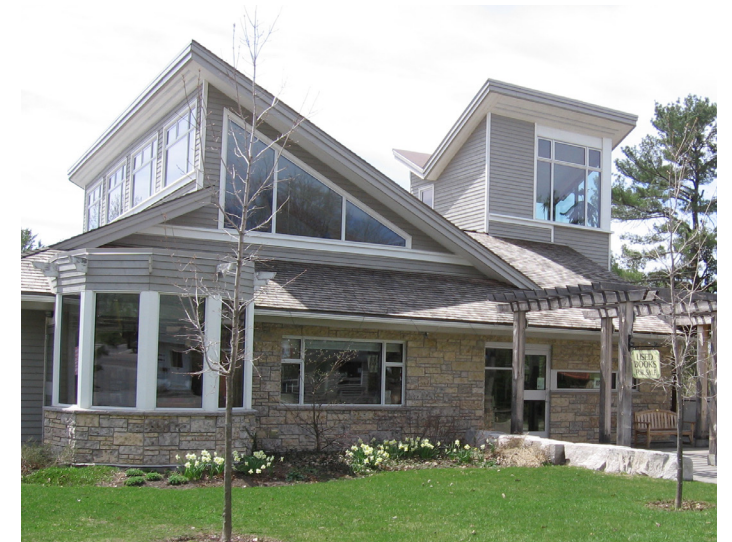
Unique and articulated massing: library building in Port Carling
